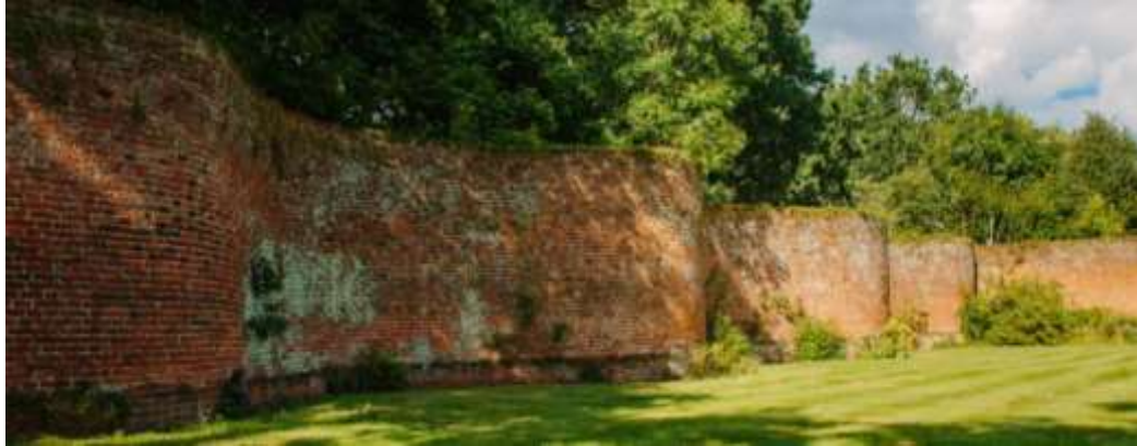
Crinkle Crankle/Serpentine Wall at West Horsley Place
